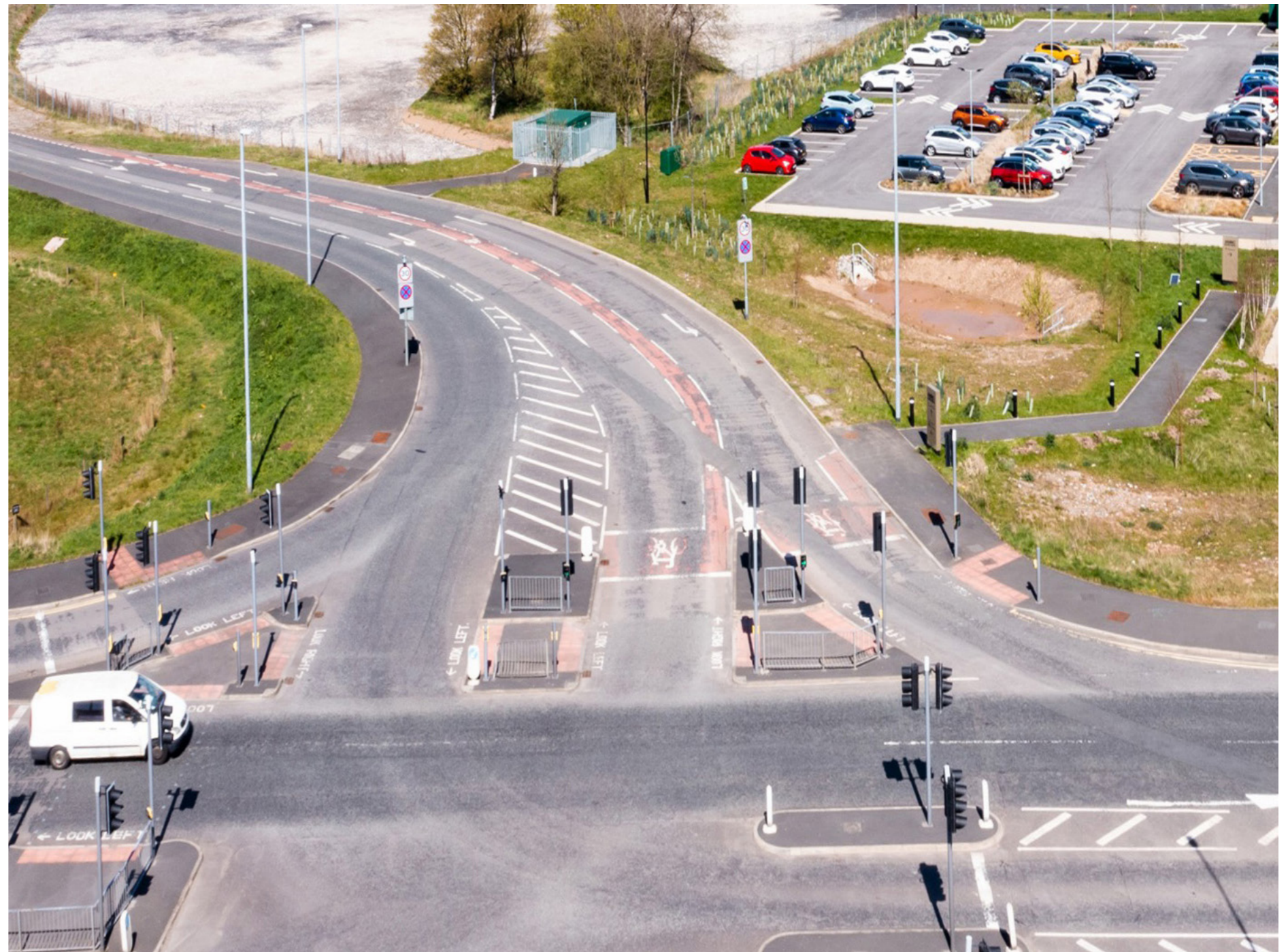
Fig. 34 - Existing photograph of the A677 junction.
